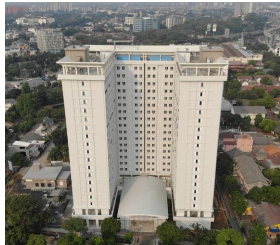
Figure 1 Pasar Jumat Apartment
