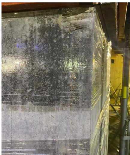
Gambar 6 Proses curing beton
